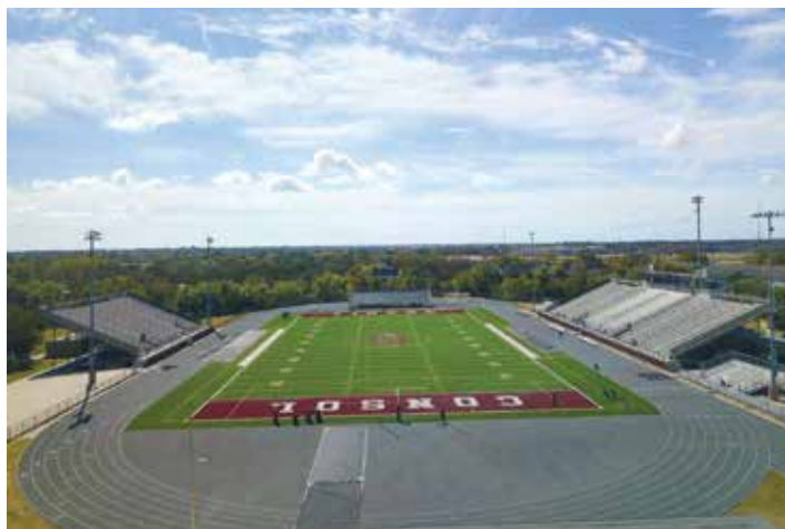
Stadium Renovations will begin Fall 2025, Baseball/Softball turfing will begin Summer 2025.
